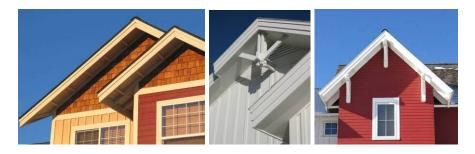
Fascia detail must have a minimum dimension of 8-inches nominal unless otherwise approved for design merit. Two-piece fascia detailing is required. Wood (including Miratec and similar products as determined by the Design Review Committee) is the only acceptable material. Vinyl or metal fascia material is not permitted. As an alternative, exposed rafter tails and entry accents are encouraged if appropriate for the architectural style.
