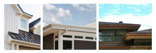
• Gutters shall be metal, and of a color and finish that blends with the finish color scheme. Gutters shall be half-round or rectangular and downspouts shall be circular or rectangular.
