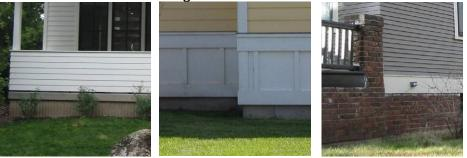
Foundation walls shall be exposed a maximum of 12-inches above the ground. Exposed foundation walls shall be built of brick, cast concrete, trimmed with horizontal members, or as otherwise approved by DRP. Concrete foundations exposed more than 18-inches above grade must have an architectural finish (texture, pattern and/or color).
